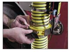
The safety disconnect coupling is to protect your investment from unexpected work place occurences, such as when a service technician forgets to remove the exhaust hose from the vehicle before moving it. The safety disconnect coupling will automatically separate to protect the vehicle and your exhaust system.
